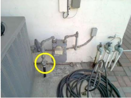
Plumbing: Gas meter and emergency shut off next to A/C unit at right/south side of house.
